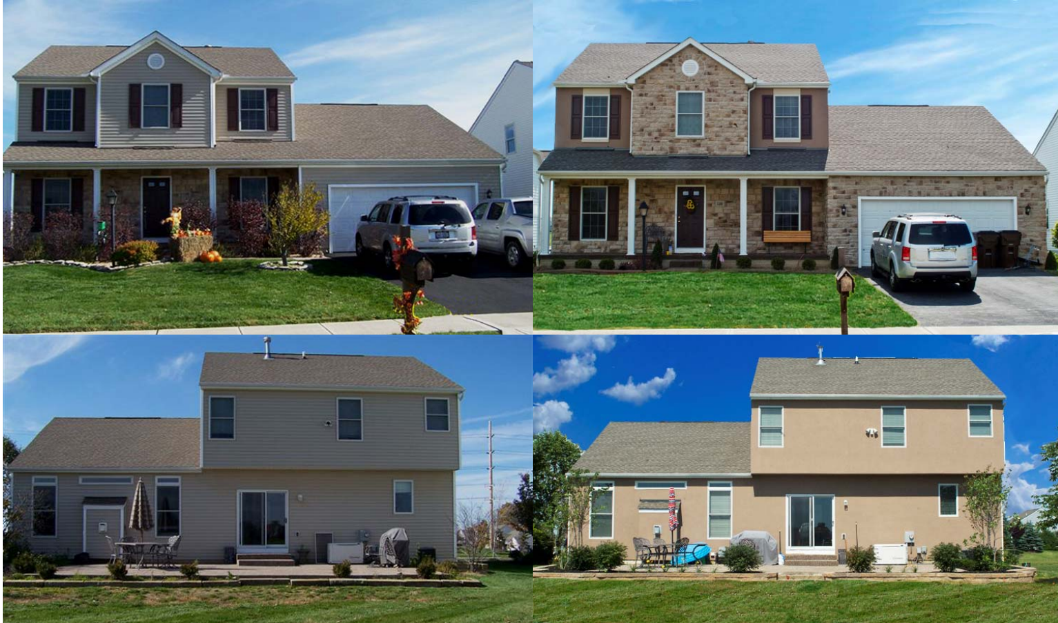
Residence Retrofit Project – Pickerington, Ohio
