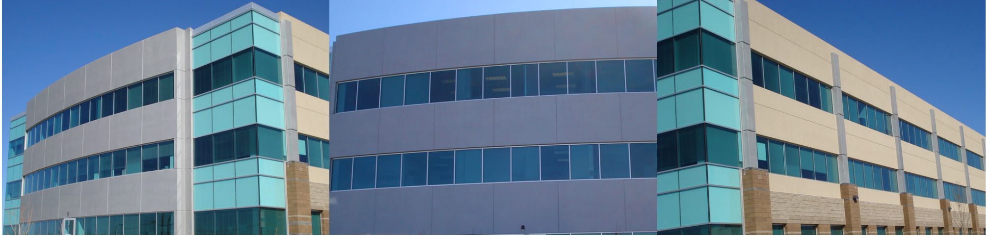
Innovation Office Parkway Center – Albuquerque, NM
